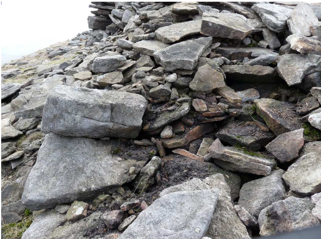
Plate 4: The photograph, taken on the eastern side of the summit, shows that there is no internal face to wall, but the infill can clearly be seen abutting the outside face.
