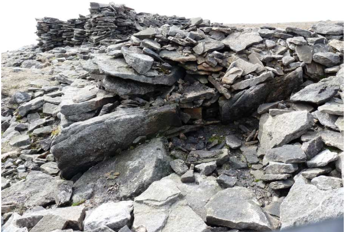
Plate 5: Orthostats forming the box sectioning of part of the wall on the north-east side of the summit.
