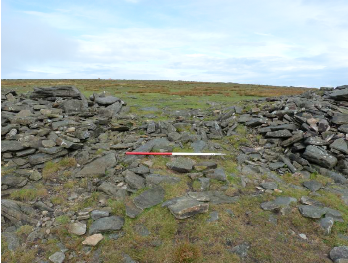
Plate 7: Showing foundation stones on either side of the entrance on south-east side of summit.
